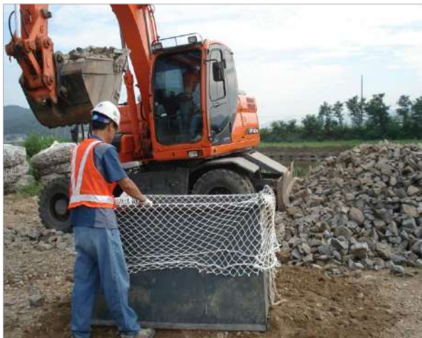
1. Putting the net over the container
