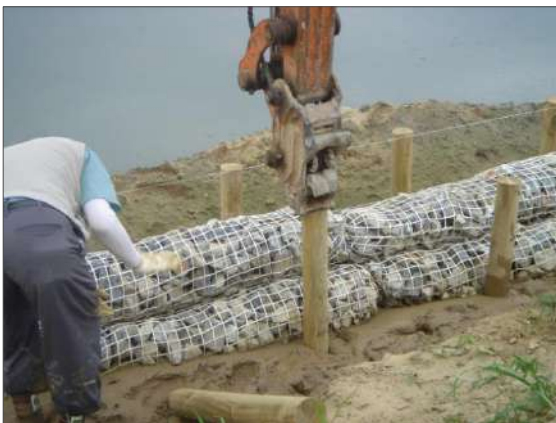
4. Installation : Pulling up, laying & fixing with antiseptic stakes(or fixing steel bar)
