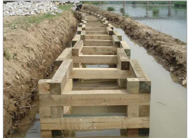
2. Stack the timber at right angles
