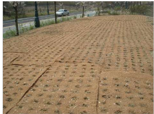
2. Installing the mulching mat
