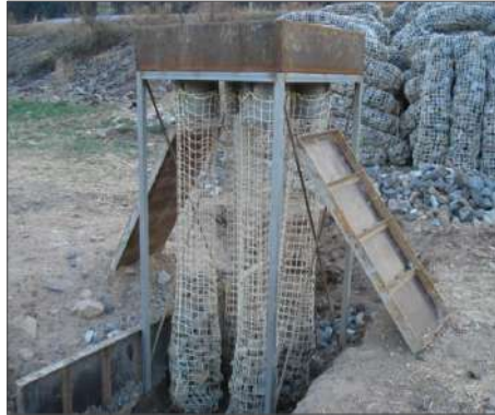
1. Install work frame 2. Mechanized in-filling work 3. Fastening the opening
