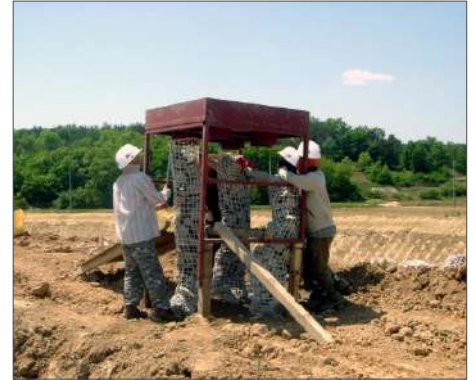
1. Install work frame 2. Mechanized in-filling work 3. Fastening the opening
