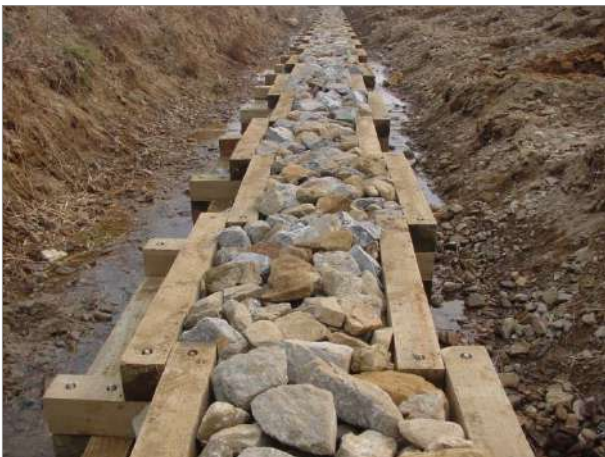
3. Filling the regular with riprap
