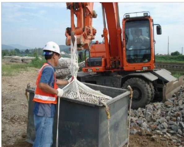
3. Fastening the opening with rope
