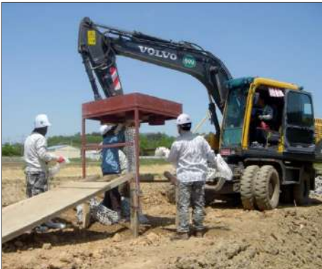
1. Install work frame 2. Mechanized in-filling work 3. Fastening the opening
