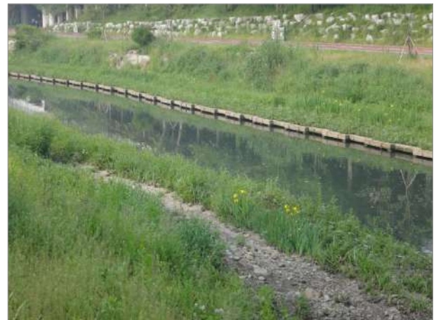
6. 10 months after the construction
