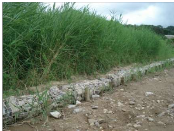
4. Installation : Pulling up, laying & fixing with antiseptic stakes(or fixing steel bar)
