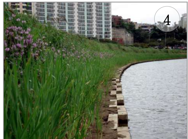
- 4 months after the construction -
