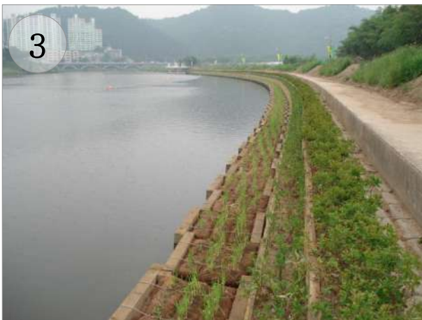
- 2 months after the construction -
