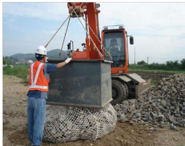
4. Pulling out the work container
