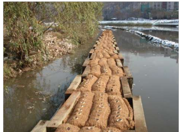
4. Installing vegetation mats
